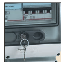
Example of lock Cat.No 0 577 35 installed on P17 unit
